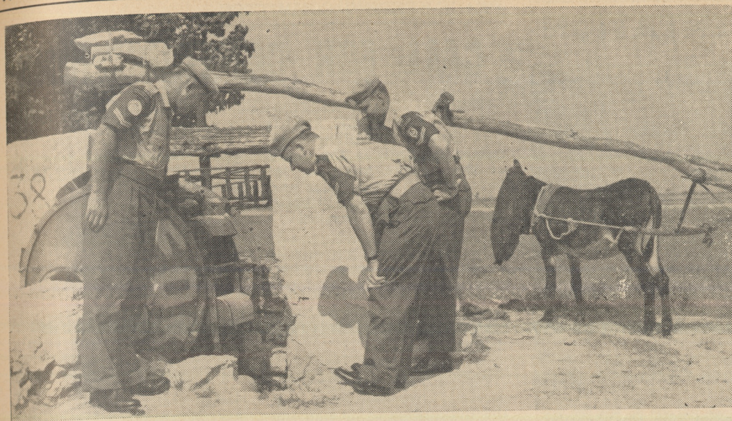
Three Corporals from the Royal Canadian Electrical and Mechanical Engineers check out mechanism of an ancient Greek Cypriot water pump, powered by a blind-folded donkey trotting round and round. The pump lifts water from a 60-foot deep well sufficient to irrigate several acres of the dry, parched ground in the north-east part of Cyprus. The three Corporals, left to right, are Jerry Marchand, Leo Fournier and Laurie Boehler.
