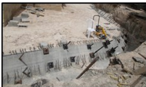
Massive ground stabilization works-micro-piling/anchoring
